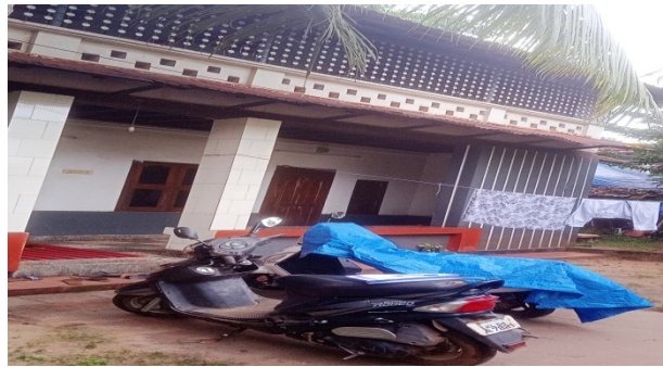
affected house in Ponnani
