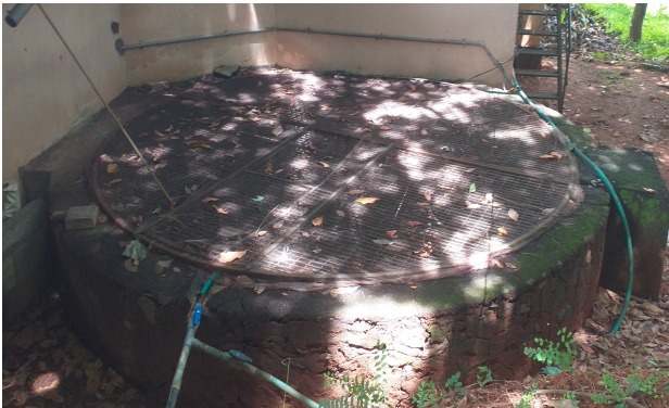
Drinking water source: affected well
