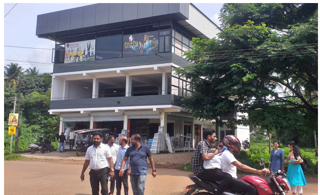
affected commercial building
