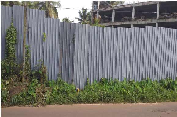
Affected under construction building
